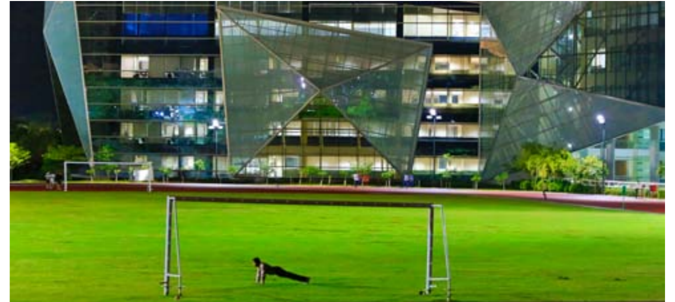
The leisure and sporting facilities at Infosys, Mysore, India, overlooked by the company offices. Infosys trains thousands of its engineers at this Global Education Centre.
